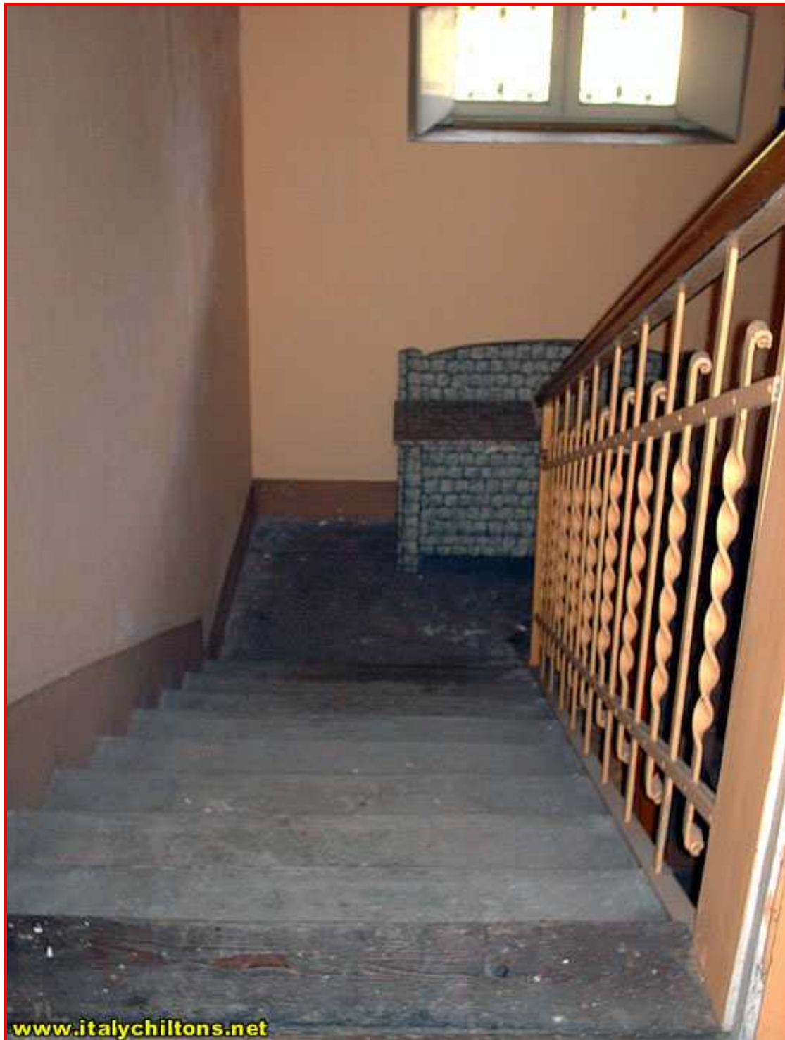
First Floor Stair Case up to Attic Loft
